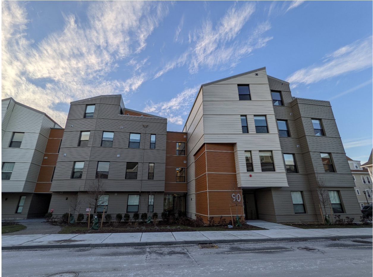
CPA funds supported the construction of UHomes, a new 20-unit homeownership development, in Allston-Brighton. 12 of the units are deed-restricted affordable condominiums, which will be available to first-time homebuyers who earn up to 80% of the Area Median Income. Source: JM Goldson
