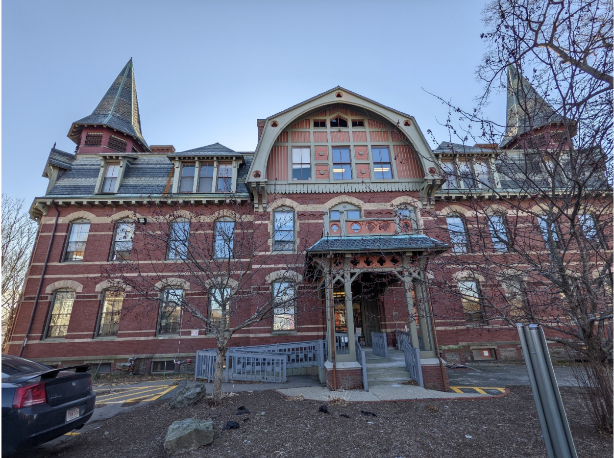
The windows of Roxbury's Dr. Marie E. Zakrzewska Building underwent restoration as part of the historic building's conversion into the Dimock Center, a residential recovery facility for men. Source: JM Goldson
